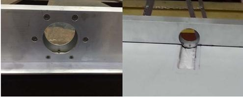
Figure 7. The PMT access point in the external frame of the enclosure
